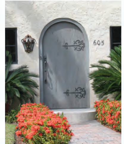
Arched plank wooden door
