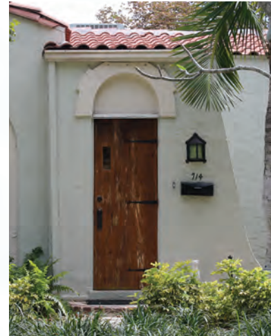
Panelled wooden door
